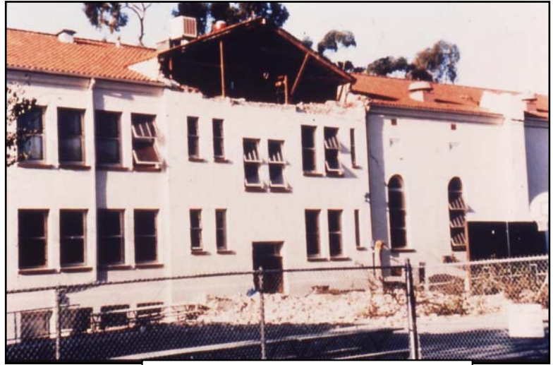
Damage to a private school in the 1994 Northridge earthquake.
