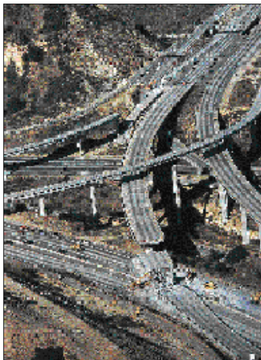
Figure 69. Two overpass collapses at the I-5/SR-14 interchange were started by failures in short, stiff columns.
