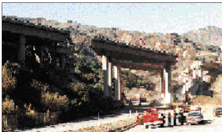
Figure 70. Deck sections fell off their seats at the Gavin Canyon Undercrossing on I-5.
